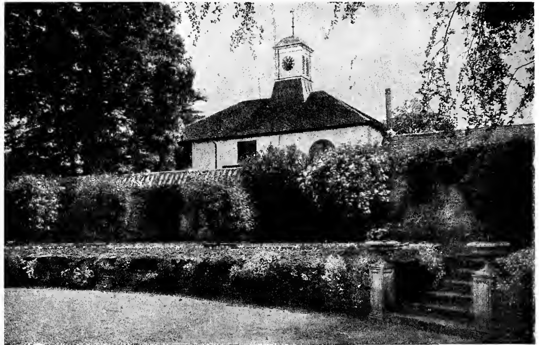
DRY RETAINING WALL IN THE ITALIAN GARDEN AT GARSTON PARK, GODSTONE.
